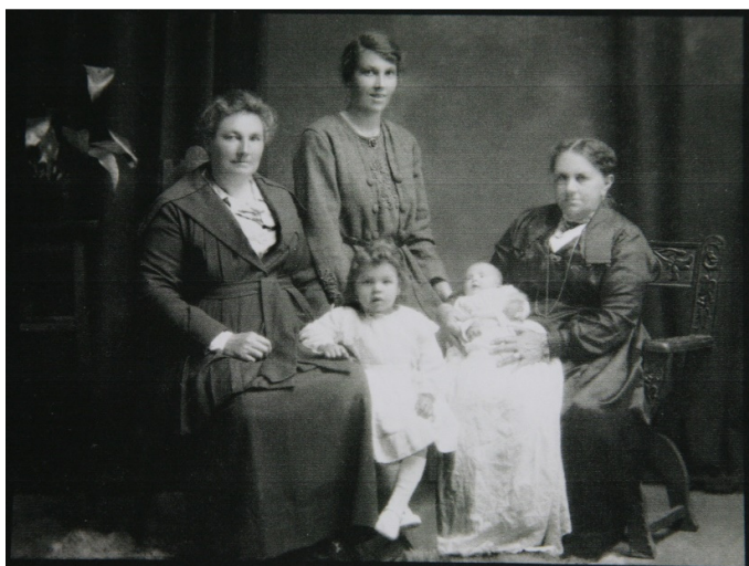
No.1 Four Generations of the Ousey / Macdonald family Box 14
